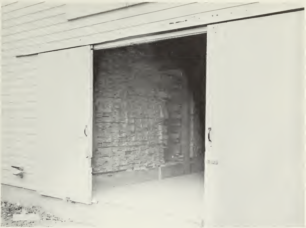
Figure 72. --Closed portion of a storage shed for lumber dried to a low moisture content.
